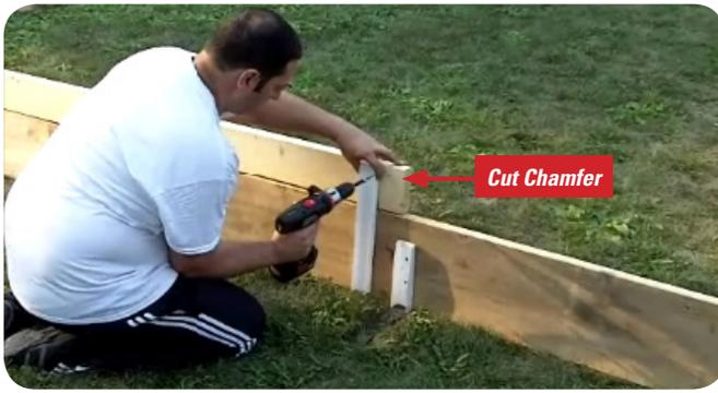
If you have a high water level or want better hockey puck retention, you will want to add a 2nd story to your rink. Attach a 2nd story using the Extension Bracket, as pictured here. The Extension Brackets can be mounted on a seam or mid-board. We also recommend you cut a chamfer on the 2nd story end board to avoid a sharp corner. When adding extension brackets, you should add more Iron Sleek Brackets for more support against the leverage. Extension Brackets are not included in our kits.
