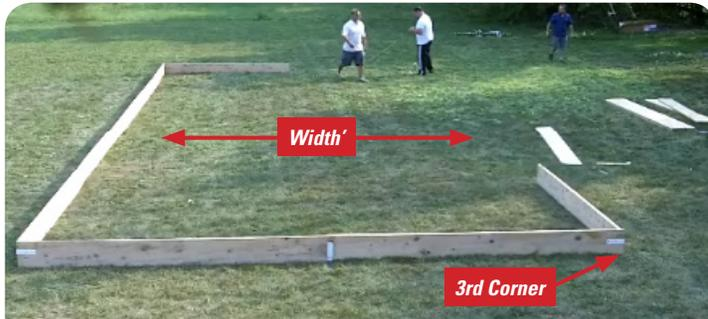
Layout the third corner and fasten an Iron Sleek Corner Bracket using the lag bolts.
