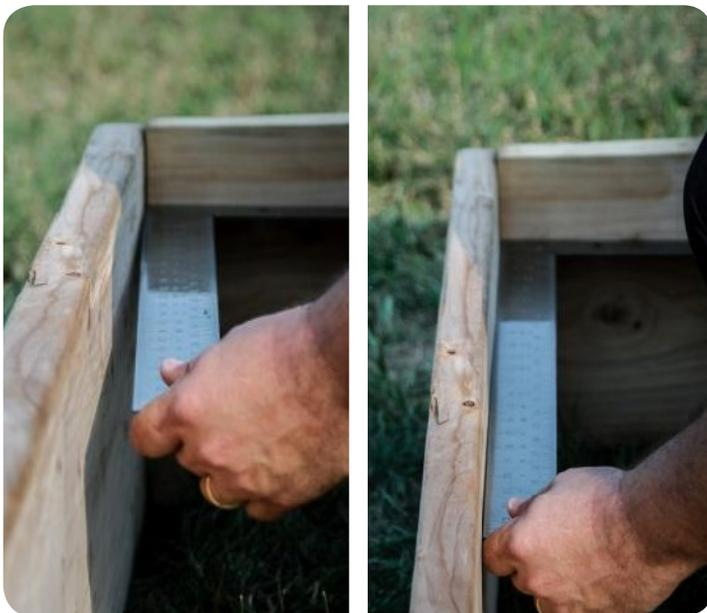
As pictured to the left, get the Carpenters Square and tuck it in the corner against the Reference Wall and the 2nd Wall, the Perpendicular Wall. For larger rinks (esp. park and recs), a Carpenters Square will not be accurate enough. You will want to use triangulation or, the "3-4-5 method". There are some great references on the web on how to use this method or give us a call.
